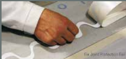
Fix Joint Protection Foil
