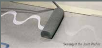
Sealing of the Joint Profile
